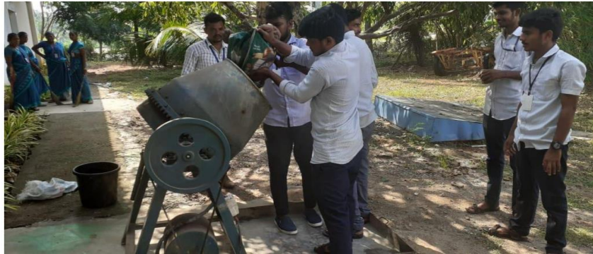
Figure 3.1 Machine Mixing of concrete
